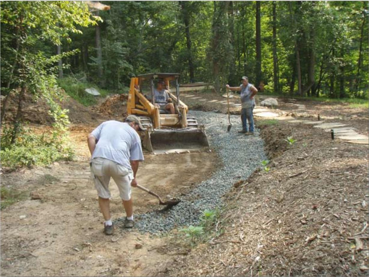
Once the drain pipes are connected to the gutter drain collection system the gravel gets consolidated and it's ready to be topped out with four inches of good soil, compost, bark mulch and water loving plants.
