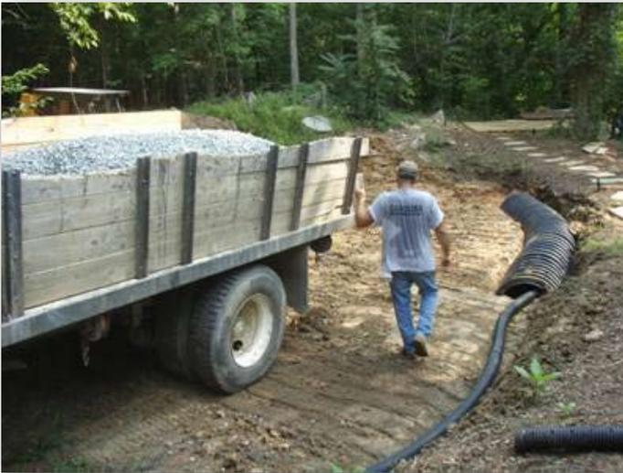
The infiltrator chambers are set into a level, flat bottomed trench dug into the bottom of the rain garden area. A berm is created to channel surface run-off into the area and 4" slotted drain tiles are used to carry gutter run-off to the infiltrators.
