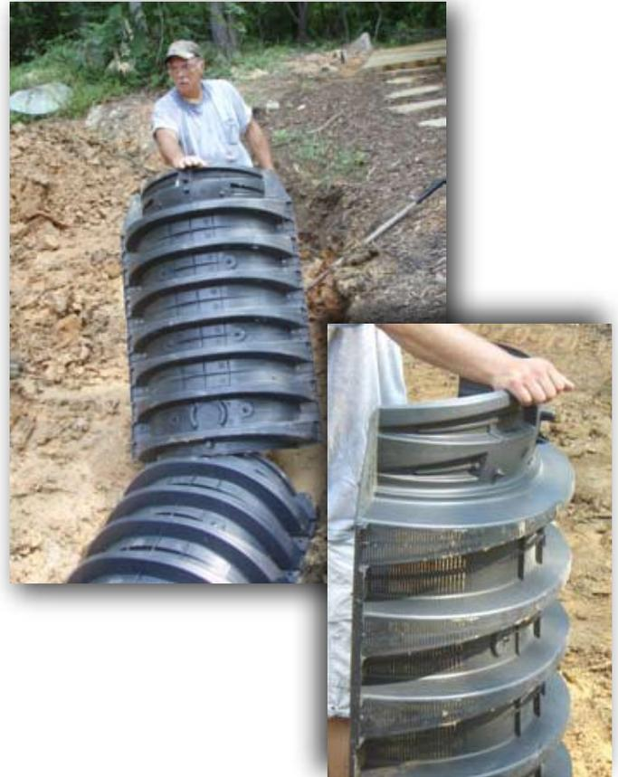
This is an “**Infiltrator**”. It’s a plastic arch about three feet wide and four feet long, it holds about 30 gallons of water and has gilled slits on the side of the ribs that releases the water to the rain garden. In this application we used five of them at \$25.00 each to create an underground water storage chamber roughly 20 feet long.
