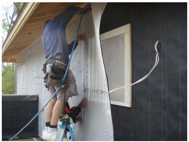
SpiderLath stands proud of the felt. SpiderLath has foam-rubber furring strips that hold the lath off the wall. Mortar easily squeezes through the lath and locks into it with a solid grip.
