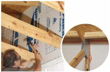
**Isolate conditioned space.** Tack OSB, Thermo-Sheath (www.fibreconverters.com), or Thermo-ply between trusses where they overhang an exterior wall. Canned spray foam is a good way to seal the sheathing in place.
