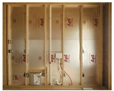
**Some interior walls might need sheathing.** Spray foam is most often applied against plywood or OSB. In some cases, such as this laundry-room wall, which will be sprayed for sound-deadening, you need to install a substrate for the foam. Here, Thermoply, an inexpensive cardboard-like material, is nailed to the studs to carry the spray foam (<a href="https://www.covalence.coatedproducts.com">www.covalence.coatedproducts.com</a>). Later, drywall will be added over the Thermo-ply.
