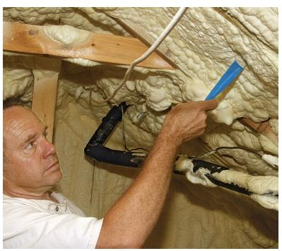
Check the foam depth before the crew leaves. Once the spray foam expands, poke it in various areas with wire to measure how deep it is. A depth gauge made of a wire flag and blue painter's tape confirms the foam depth. The wire is so thin that the hole it leaves will not affect the foam's performance.
