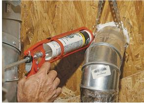
**Seal penetrations with caulk.** Expanding spray-foam insulation will find its way through any crevices larger than 1â,,8 in. Caulk around pipe penetrations before the spray foam arrives to keep it from seeping onto the siding.
