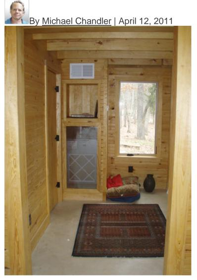
This 640-square-foot cabin with radiant floor and spray foam insulation hardly needs any cooling, but it needs dehumidification provided by the 11,700 BTU/h vertical PTHP that fits in the bottom of the display cabinet. At 10.7 SEER, its doesn't meet code minimums despite the efficiency of the envelope. A little unit like this would be perfect for a number of superinsulated situations, except it's illegal.
