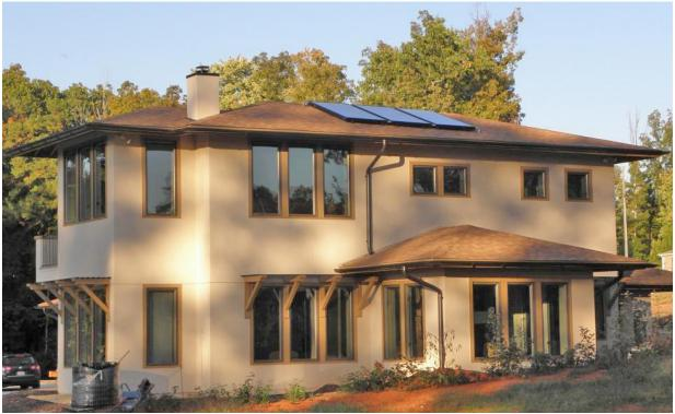
Wide (37 in.) roof overhangs and lattice shade structures protect windows from the summer heat. The three roof-mounted solar collectors are connected to a 180-gallon storage tank which supplies hot water to the radiant floor. Image Credit: Michael Chandler, Chandler Design-Build
